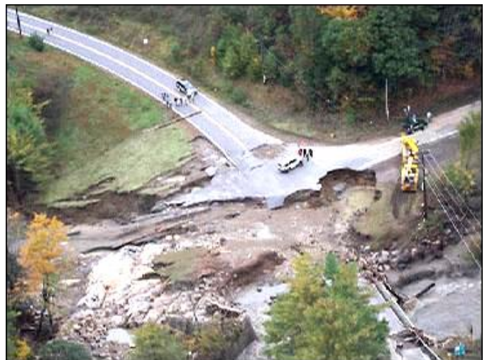
Washed out road in SW New Hampshire, October 2005
