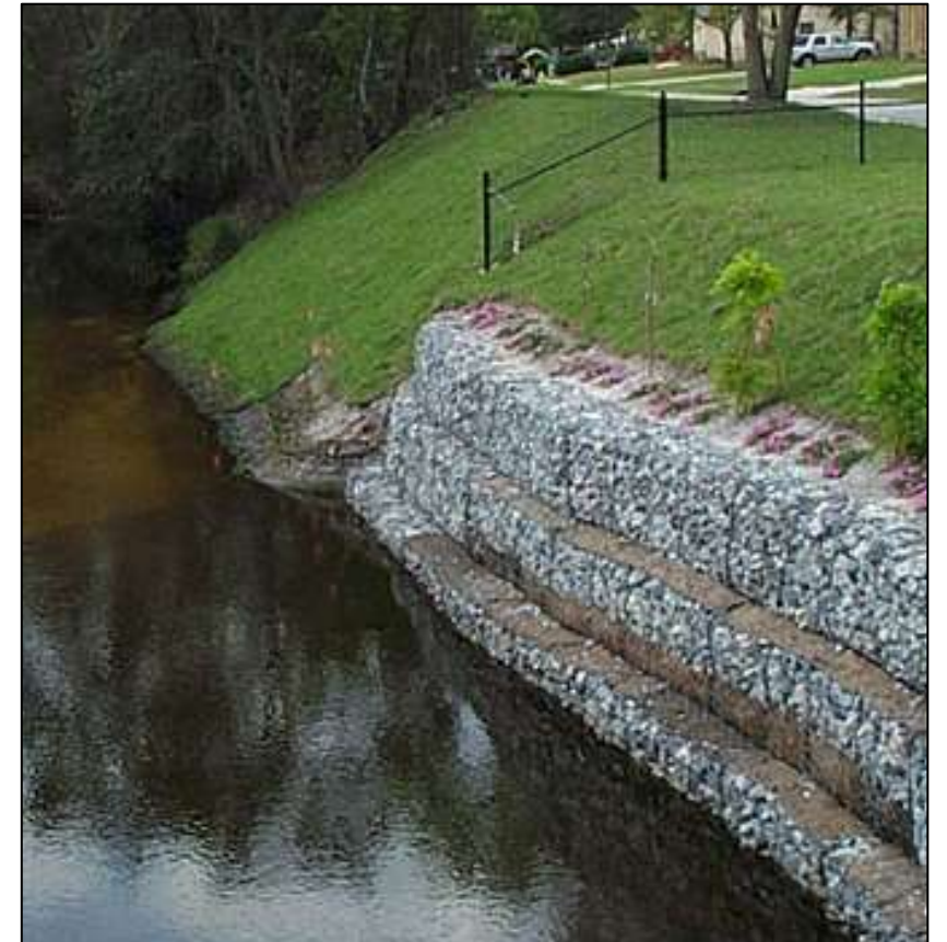
Gabion baskets in use
